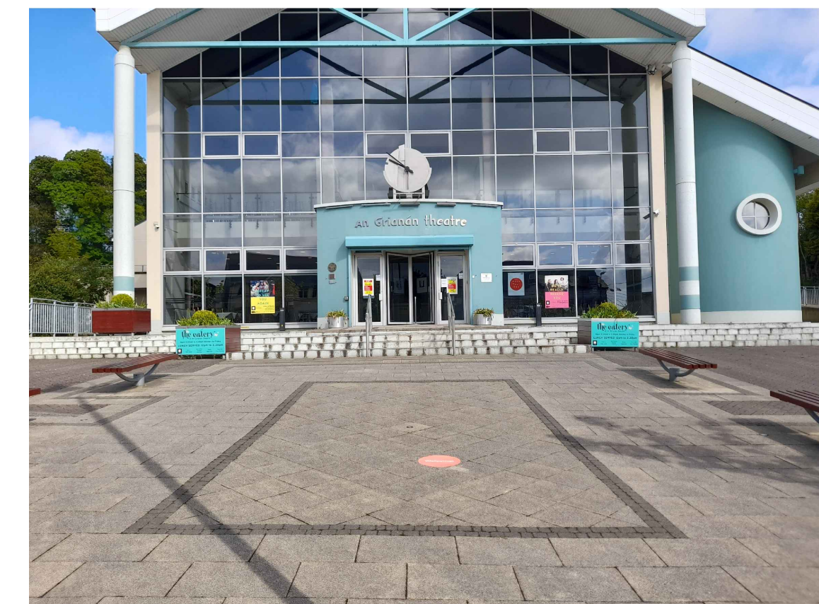
Existing square and theatre facade
