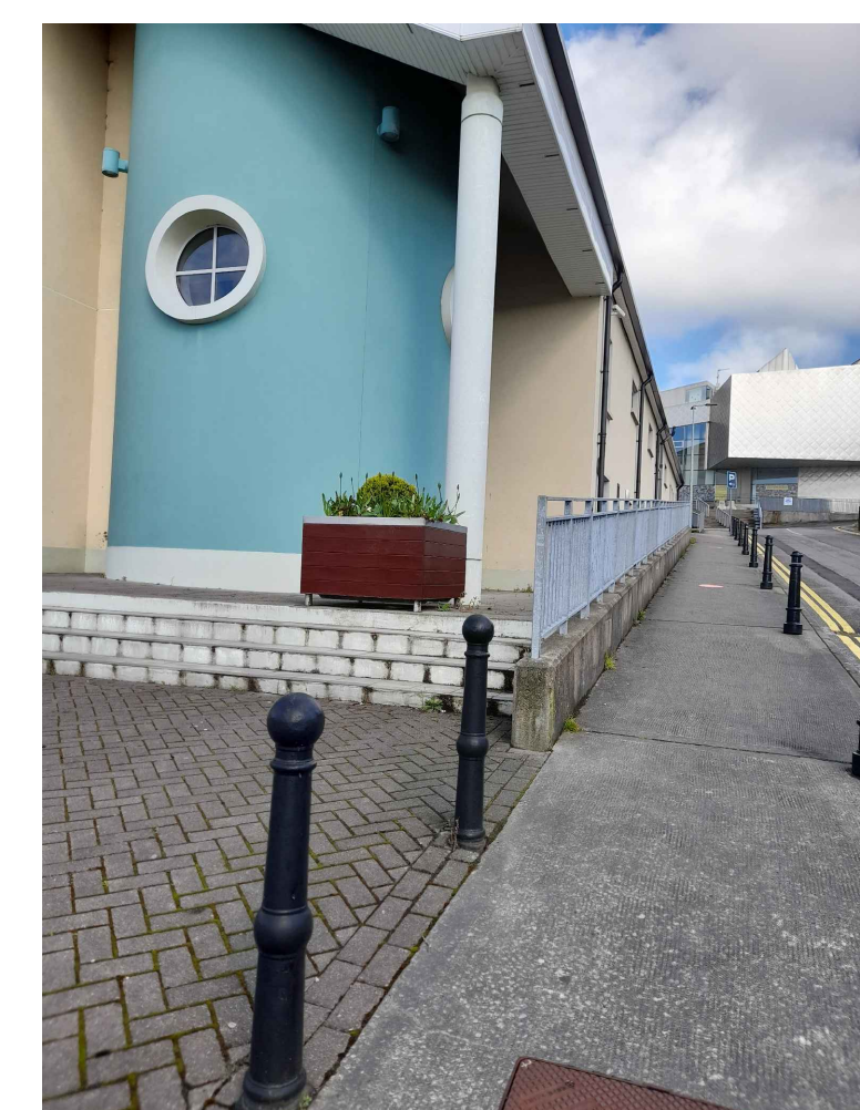
Pavement East of square
